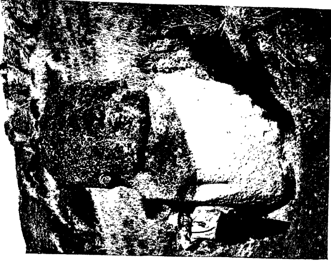
Showing scamped work in lower part of figure, no right hand curved, and surface only coarsely chiselled. [No. 36. Fig. 47.]
